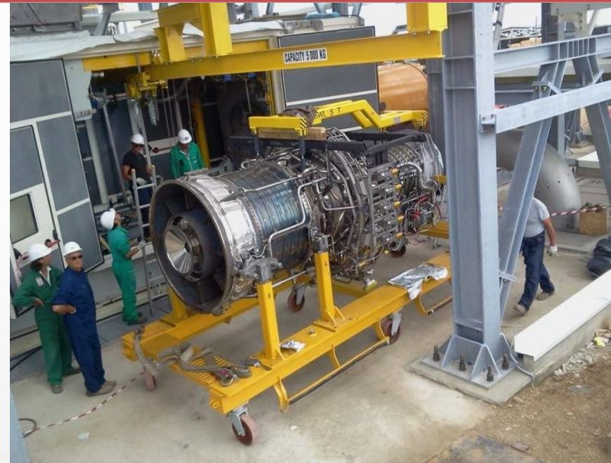
Project: Gas compression station 2 x 30 MW turbo compressors, Messina, Italy
