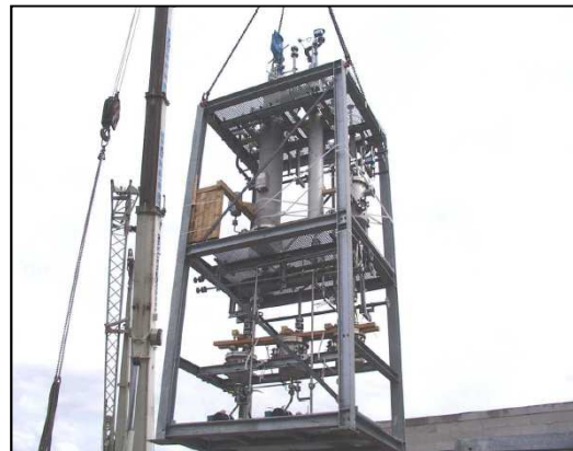
SKIDS ERECTION
